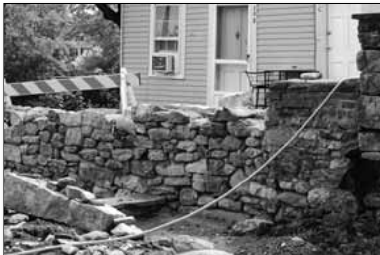
The old stone foundation that was once part of the Holley Block, in Bicentennial Park, was repaired this year.
