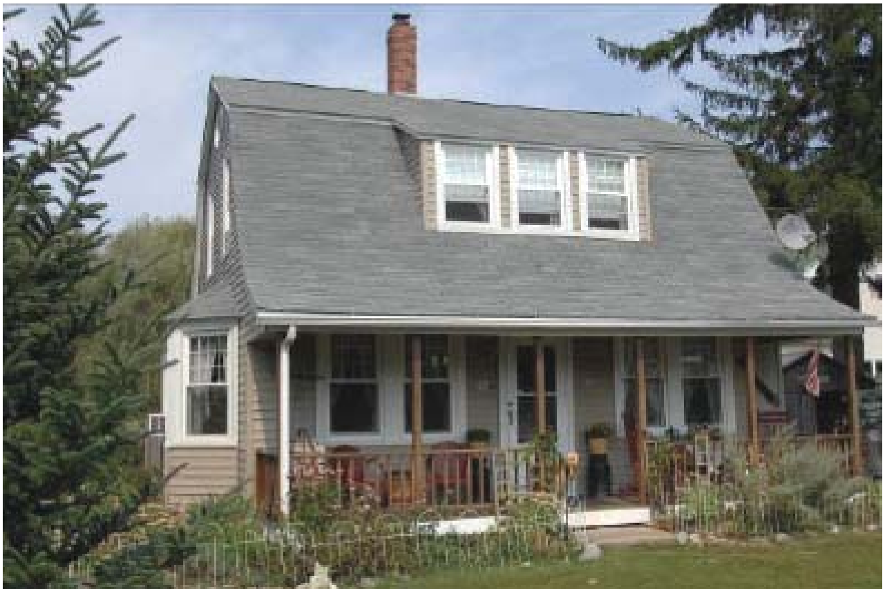
Single Family - Renovation Cornwall Housing Corporation Cornwall, CT
