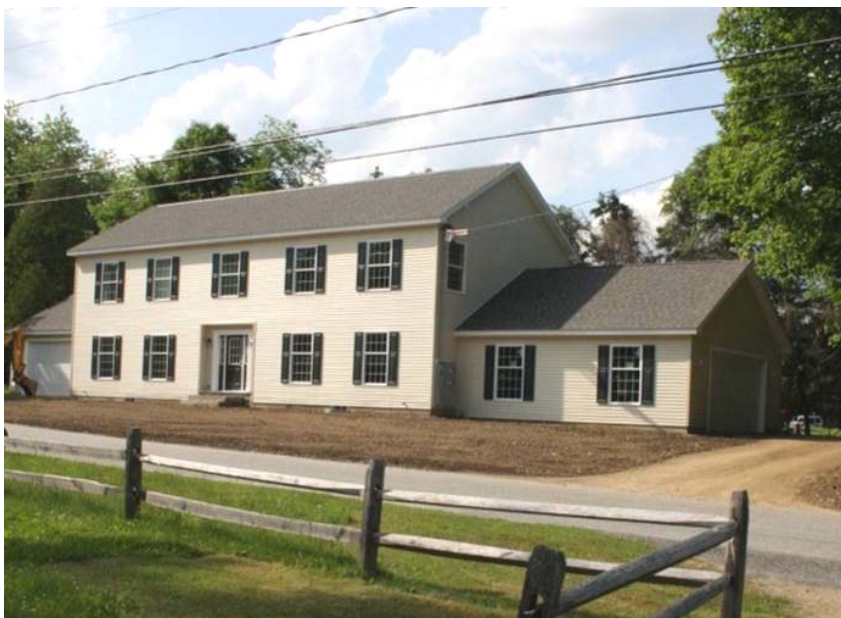
Duplex - Under Construction Salisbury Housing Trust Salisbury, CT
