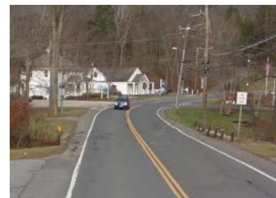
Figure 8. Inadequate Guide Rails
