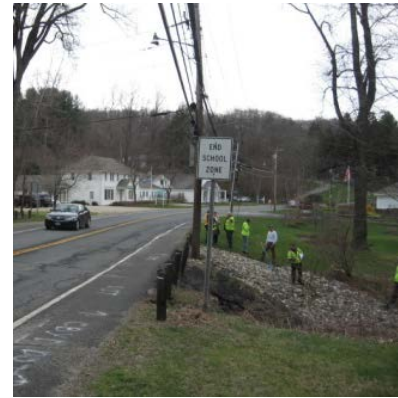
Figure 7. Eroding Roadway at Culvert
