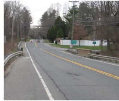
Figure 10. Narrow Bridge Crossing
