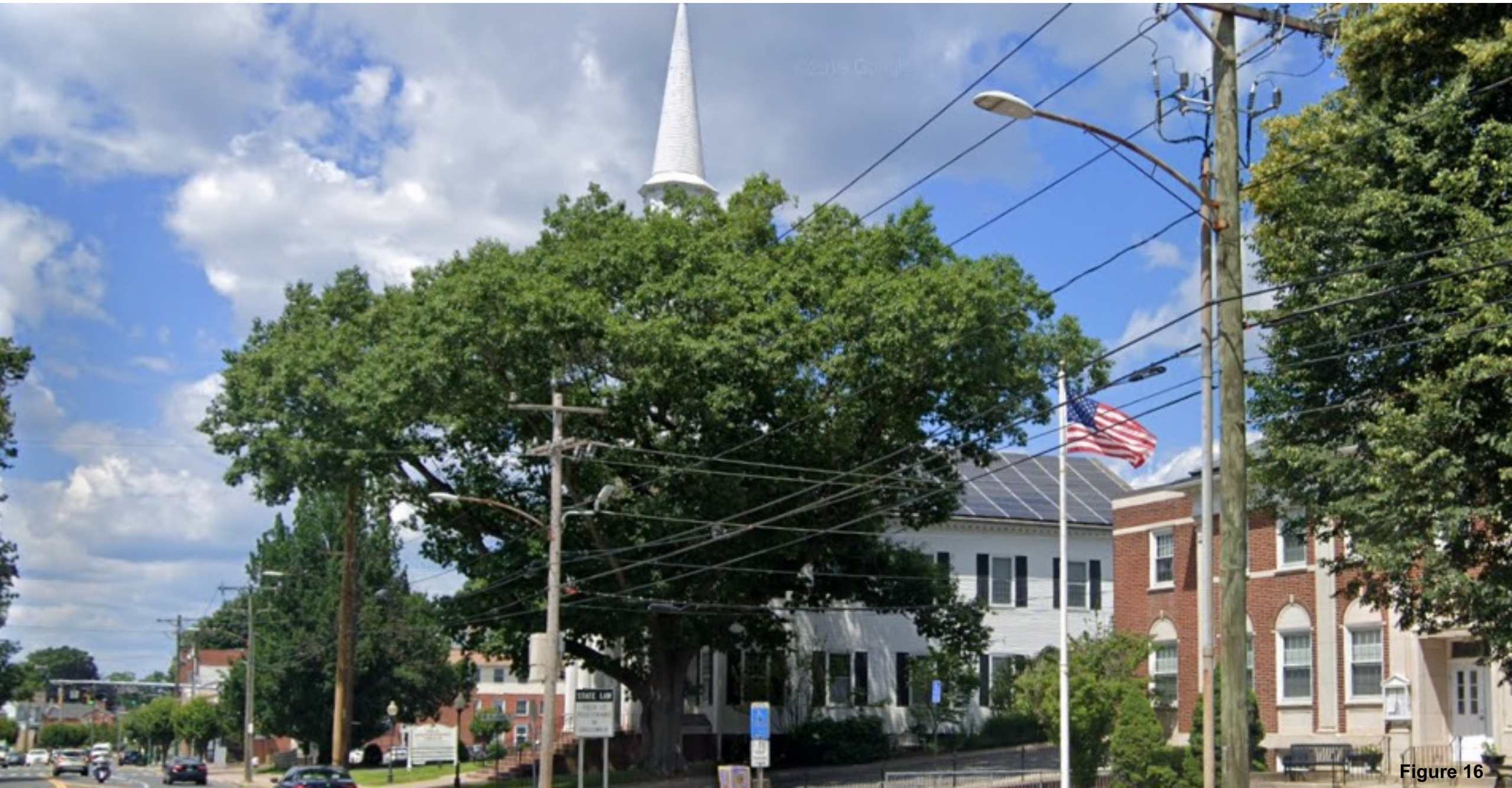
Example of Existing Solar on Church Roof – First Congregational Church of Southington
