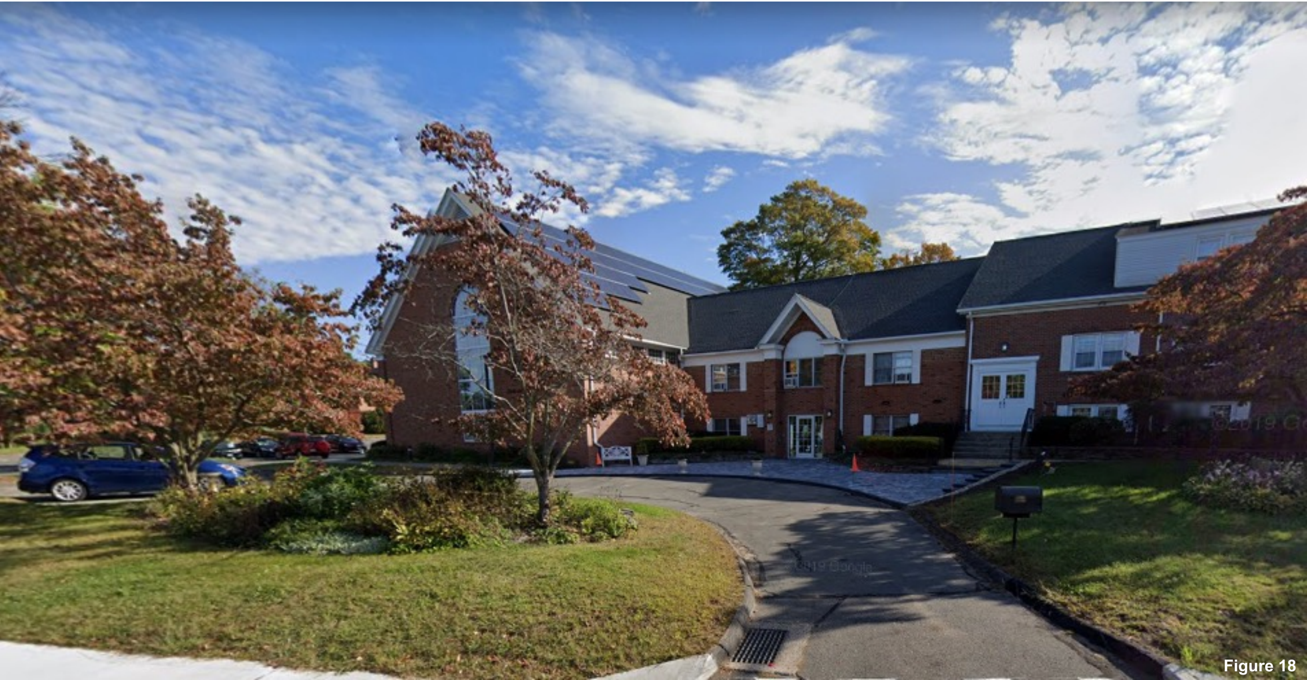
Example of Existing Solar on Church Roof – Wapping Community Church, South Windsor
