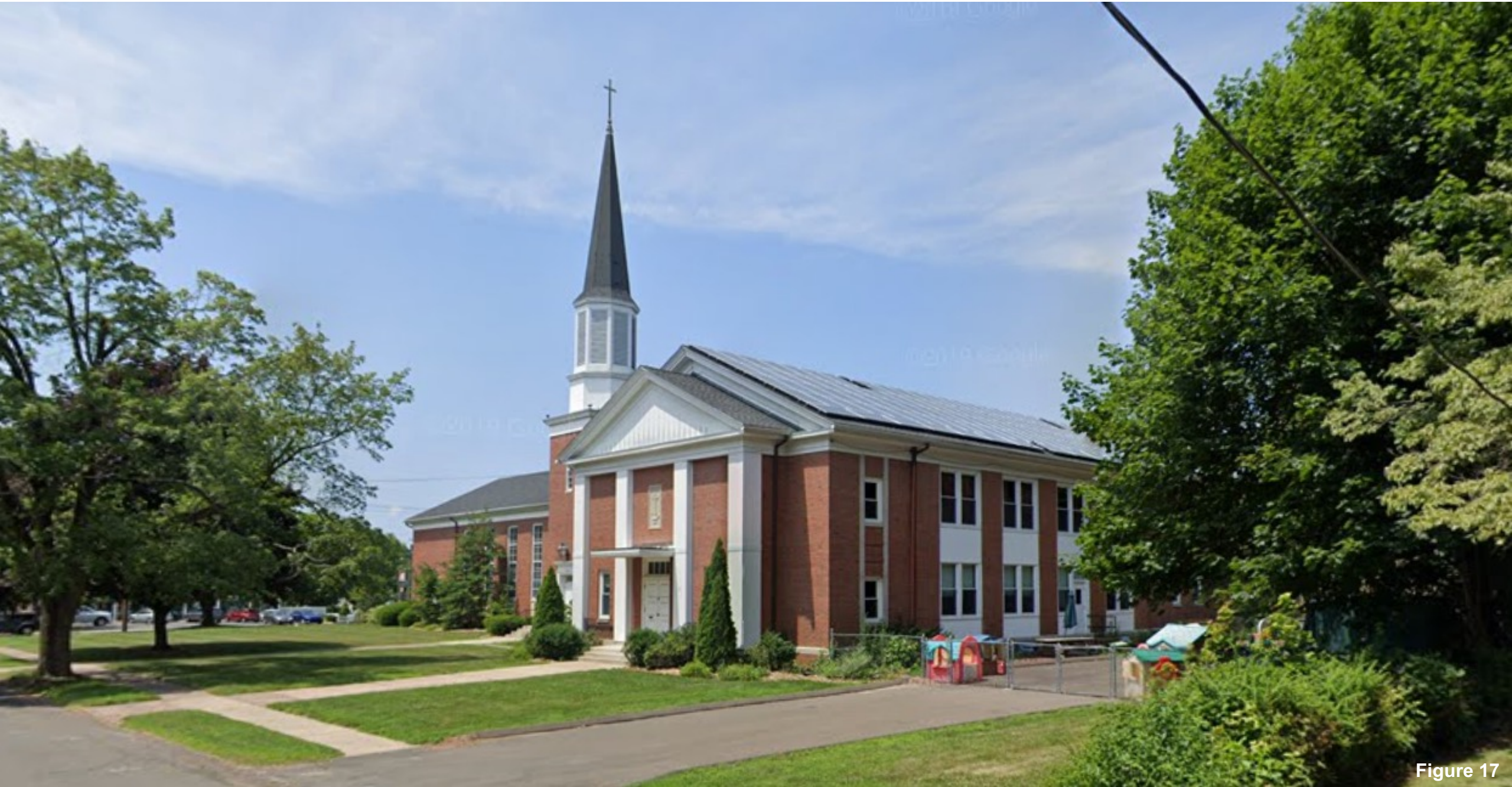
Example of Existing Solar on Church Roof – Spring Glen United Church, Hamden
