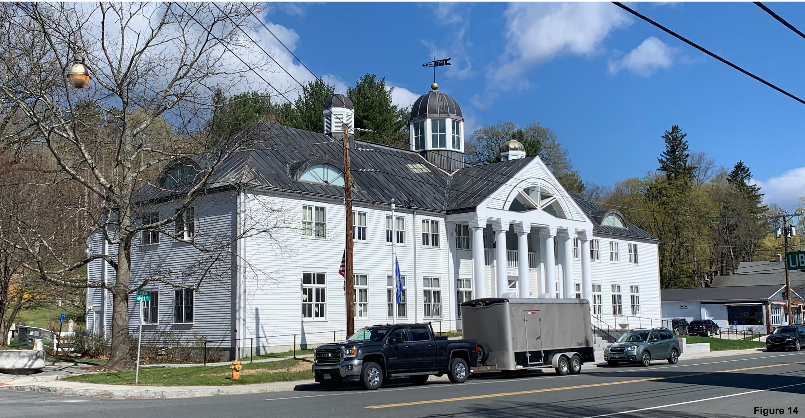
Example of Existing Local Metal Roof – Salisbury Town Hall
