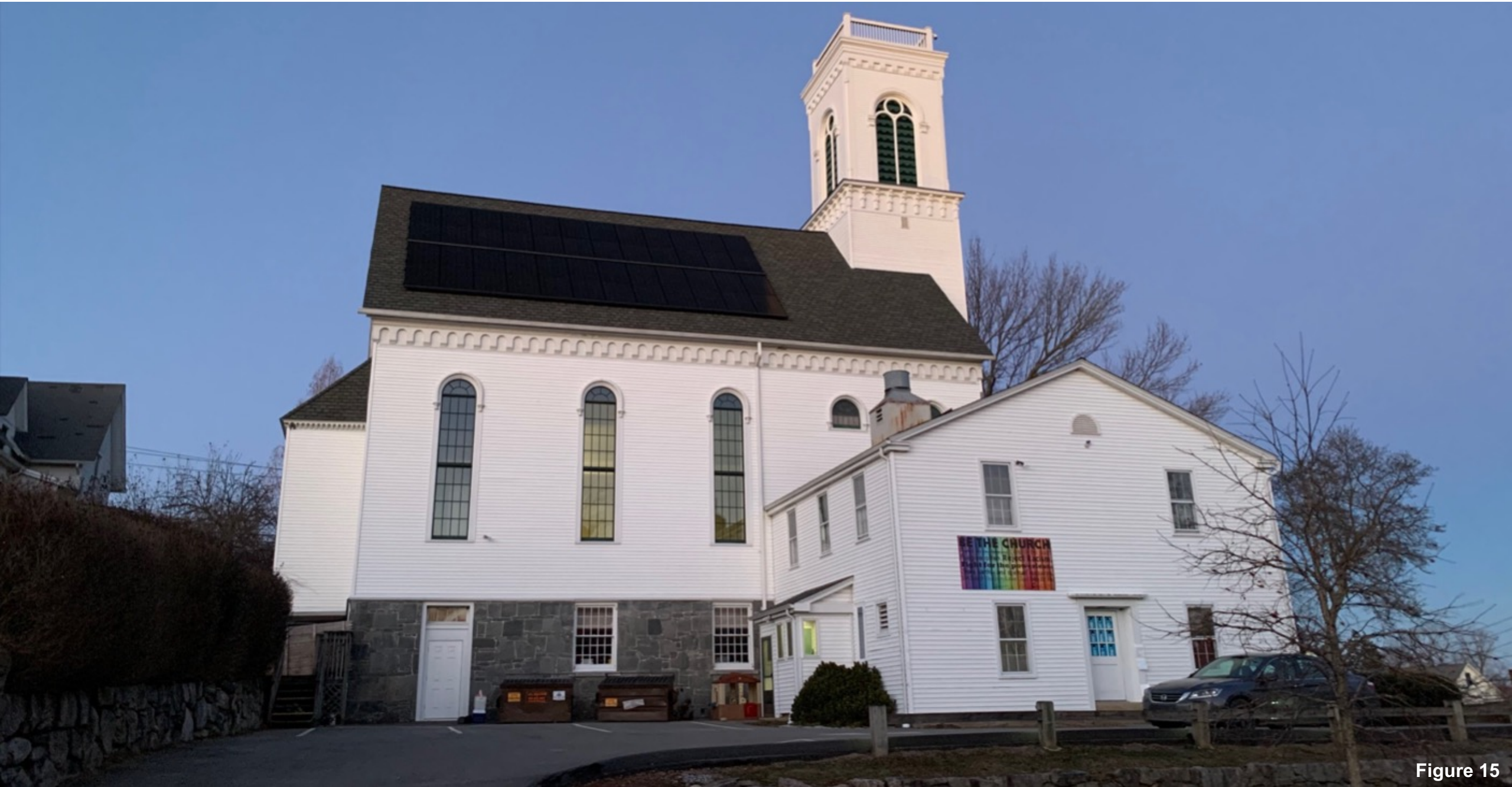
Example of Existing Solar on Church Roof – Essex Congregational Church
