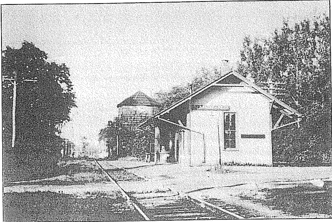
Salisbury station and water tower at Library Street.
