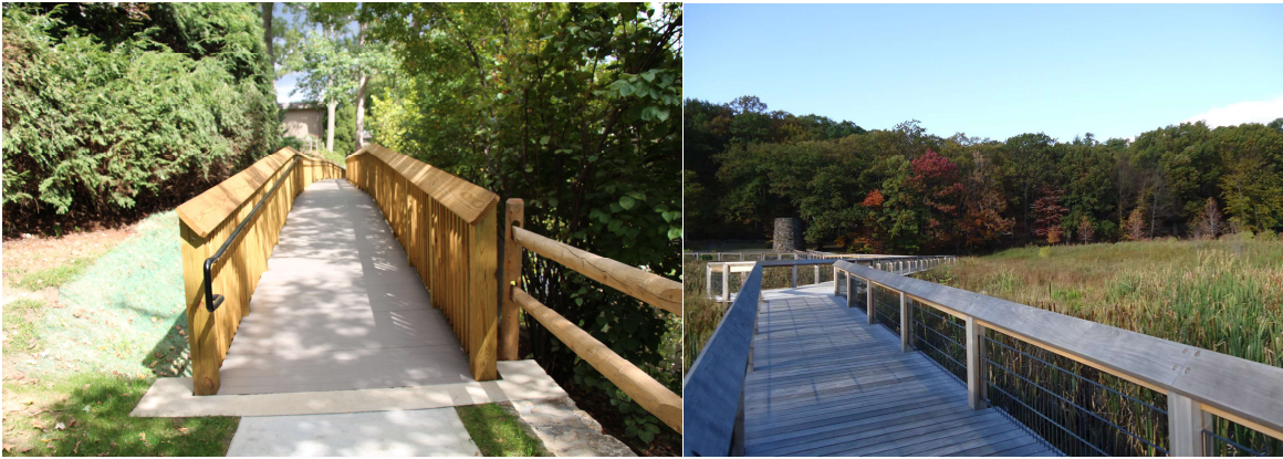
Left: Composite Decking with Timber Railing; Right: Ipe Hardwood Decking and Steel Mesh Panel Railing
