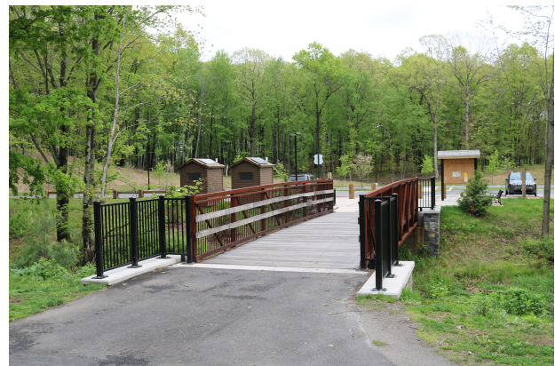
Prefabricated Steel Truss Bridge – Weathering Steel and Ipe Hardwood Decking
