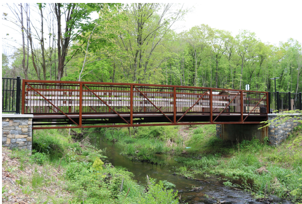
Prefabricated Steel Truss Bridge – Weathering Steel and Ipe Hardwood Decking
