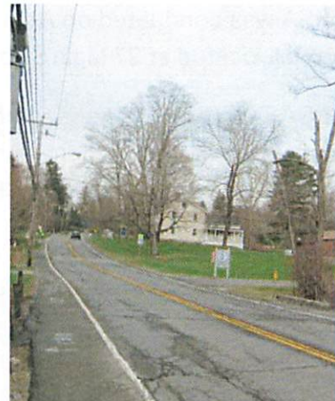
Figure 5. Deteriorating Pavement
