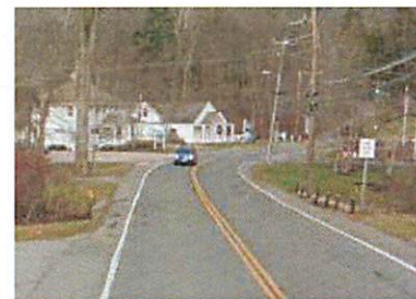
Figure 8. Inadequate Guide Rails
