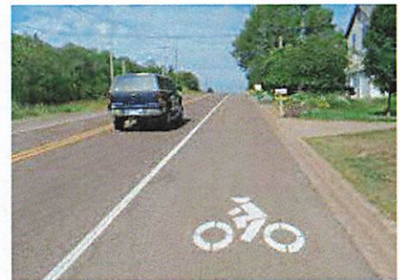
Figure 11. Typical Bicycle Lane
