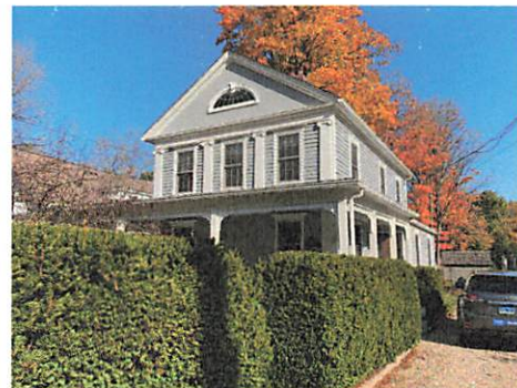
A gable-front Federal-period house on Main Street, Salisbury Village, with an unpaved drive and rear outbuilding. The house's attic fan is a distinctive Salisbury design, characteristic of its period. The Ionic pilasters with carved Ionic volutes on the façade are a characteristic classical touch.
