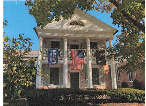
A gable-front house in the Federal style, 8 Main Street, Salisbury Village, built of brick. A triangular gable pediment, trimmed with a modillion course, and simple roof profile enhance the building's dignified aspect. (Yet another distinctive gable fanlight.)
