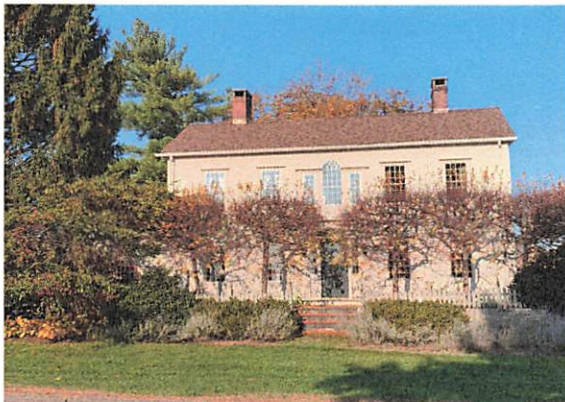
No. 158 Lime Rock Road, early 1800s, is a five-bay center-hall house with a Palladian window.
