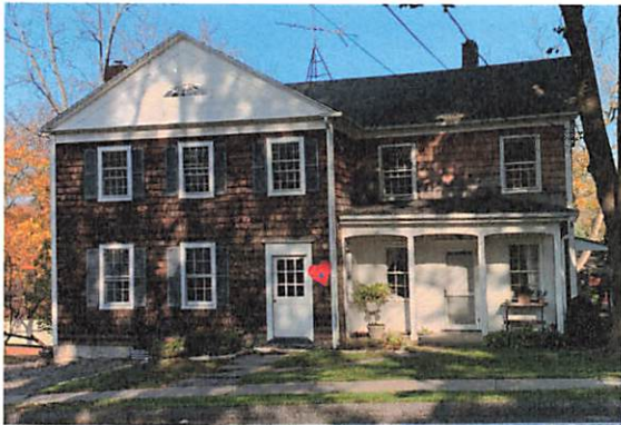
28 Sharon Road, Lakeville: A vernacular Federal-period house with a wood-shingle exterior. The building has a typical composition of two intersecting gabled sections.
