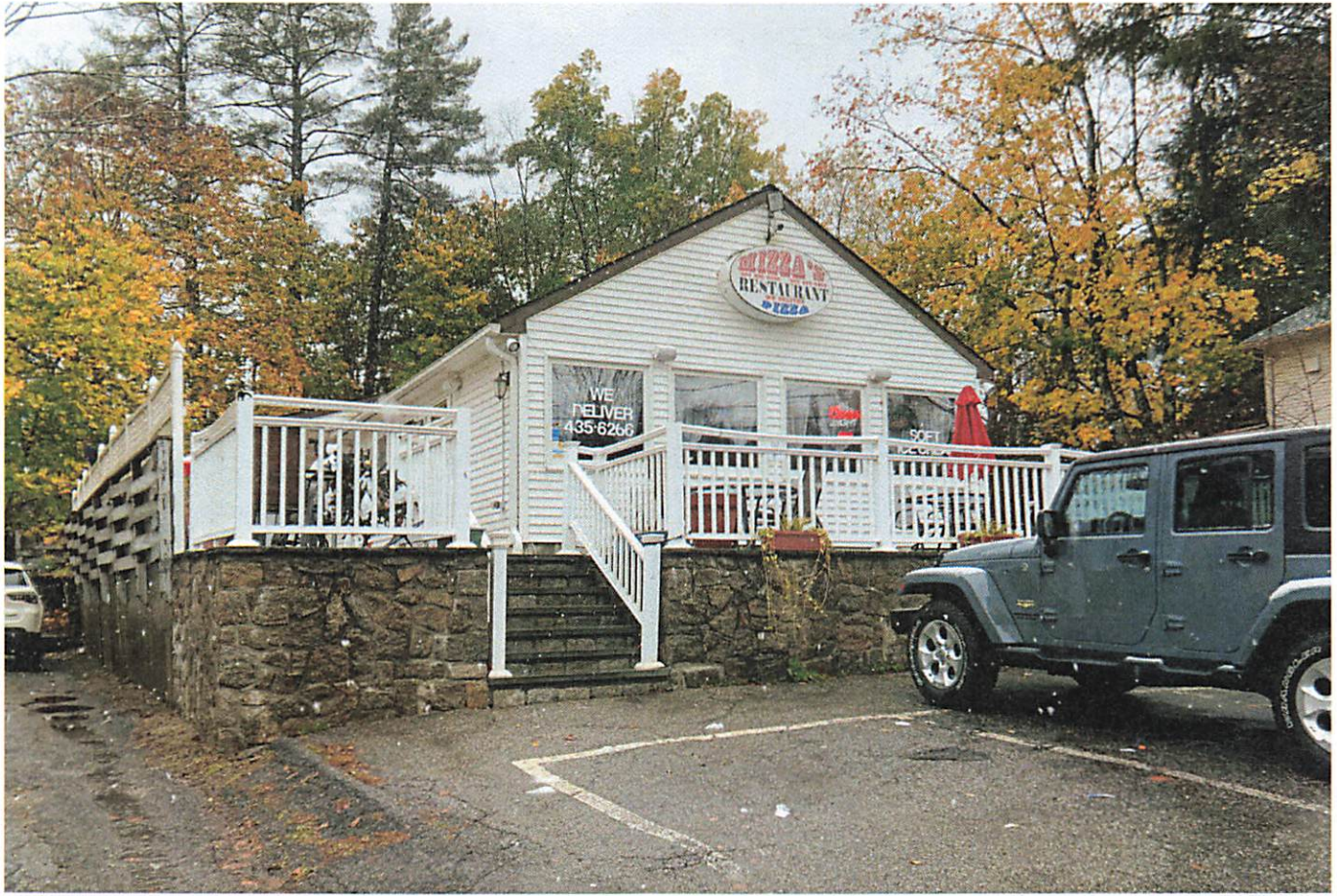
To support the fact that large 3 story buildings are common in the area, this is the front of the building on 27 Elm Street.
