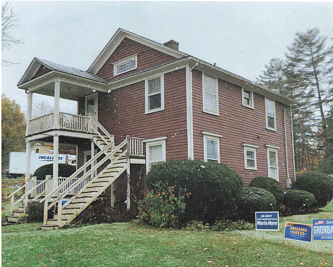
Building on Rte 41 near intersection with 44
