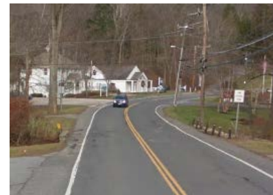
Figure 8. Inadequate Guide Rails
