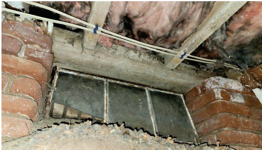
7. Floor joists supported on wood sill plate bearing on brick wall on top of foundation wall.
