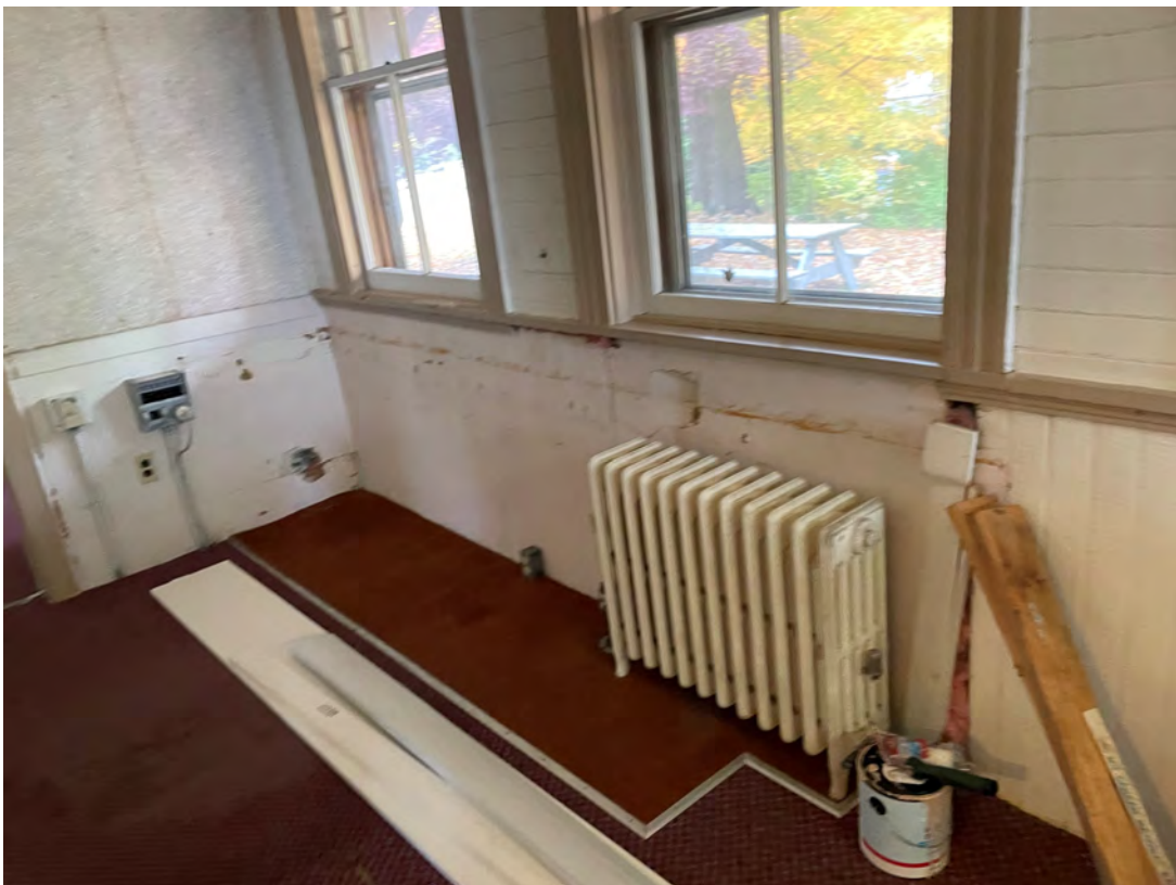
Figure 3 - Cast iron radiator & Generator Fuse Panel
