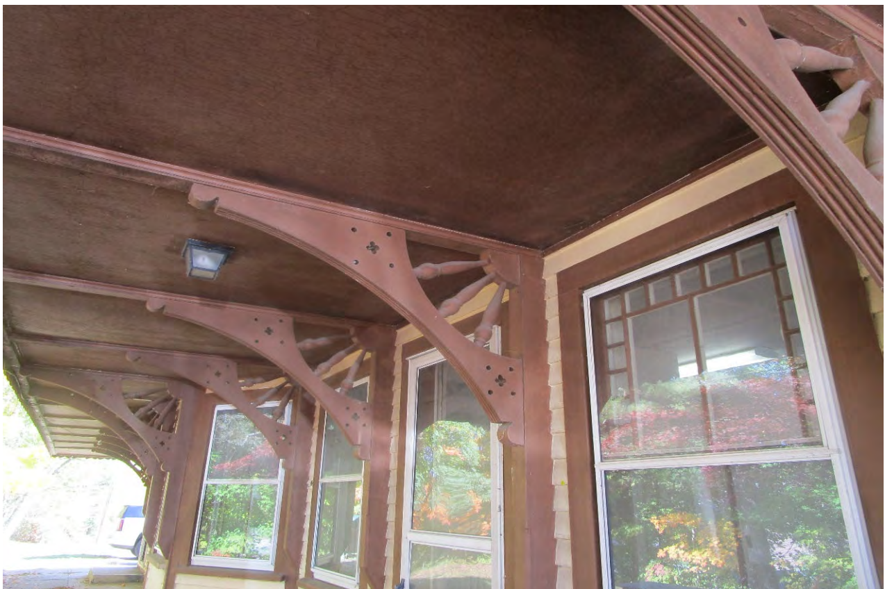
13. ROOF OVERHANG AND ROOF BRACKETS.
