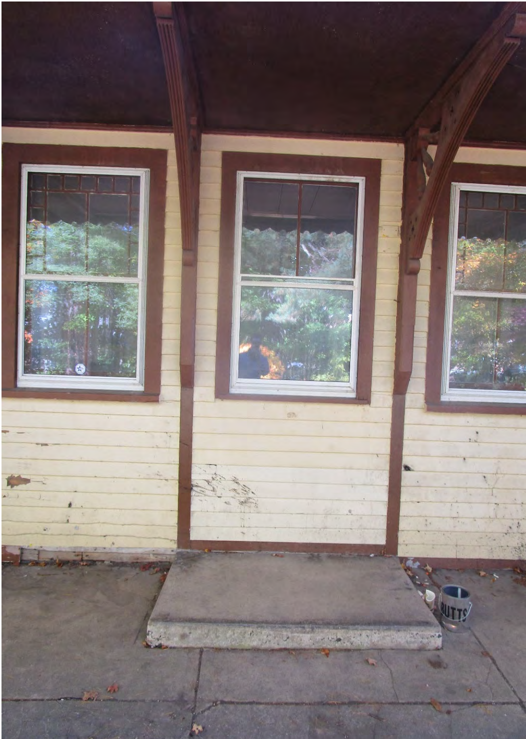
19. NORTH ELEVATION INFILLED OPENING.
