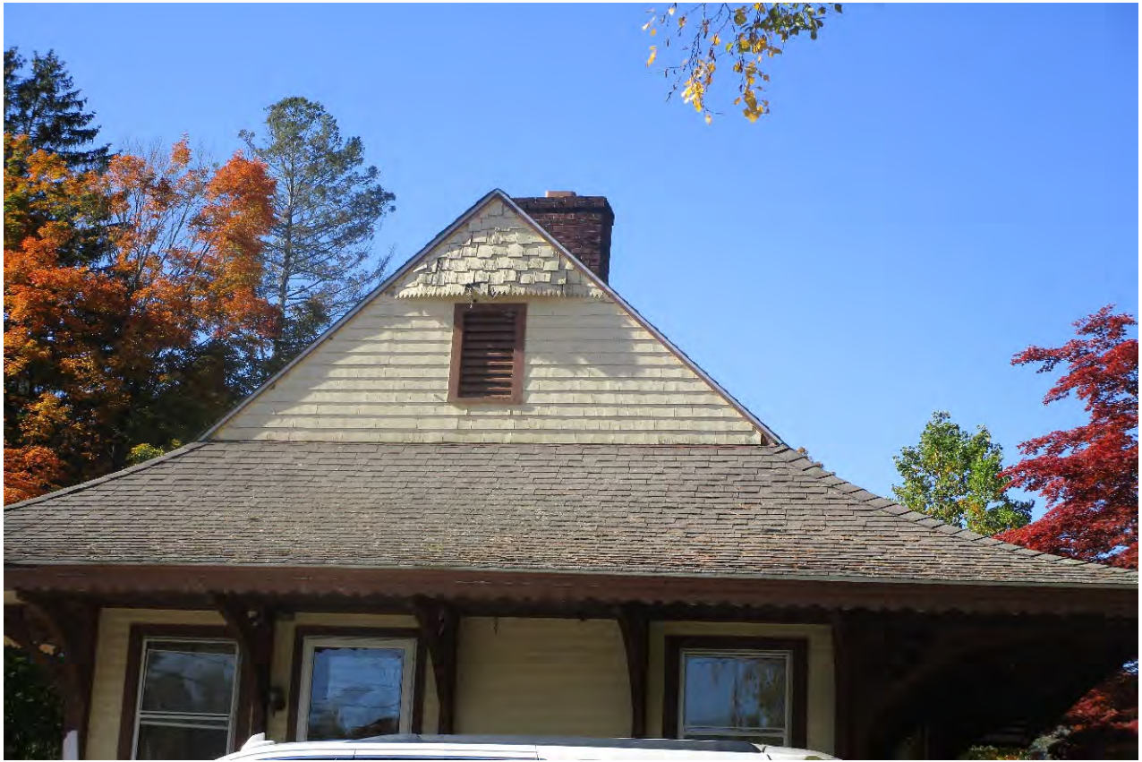
10. WEST ELEVATION ROOF GABLE AND LOUVER.
