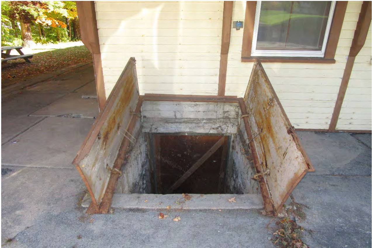
23. WEST ELEVATION BULKHEAD BASEMENT DOORS.
