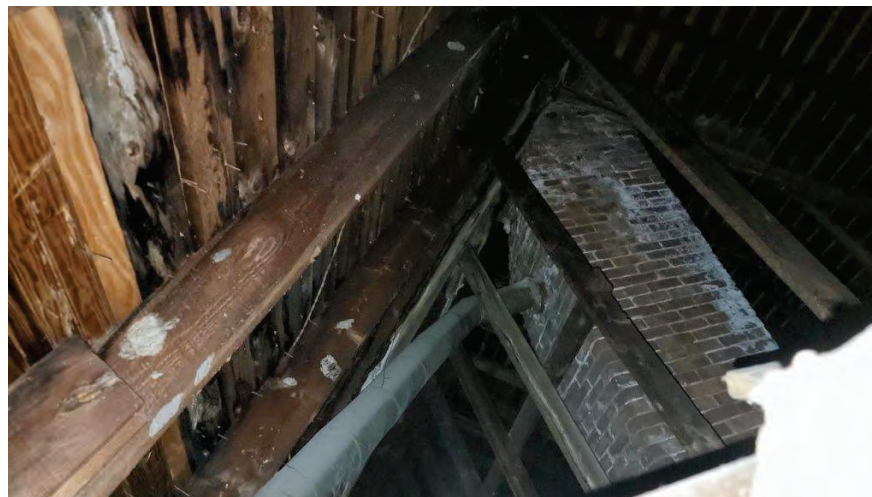
18. Limited view of roof framing. New plywood visible between original furring.
