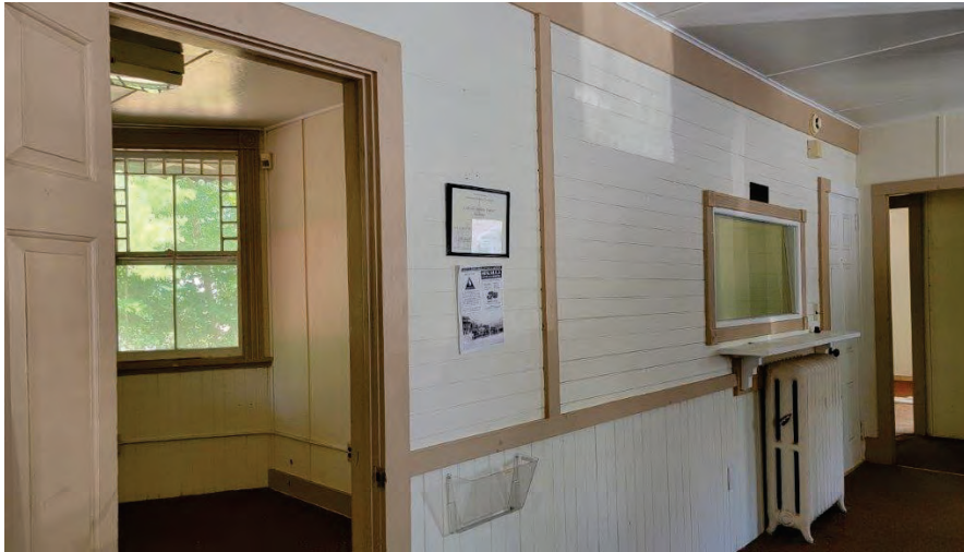
13. Interior walls may be supporting ceiling loads. Investigate before removing or altering.
