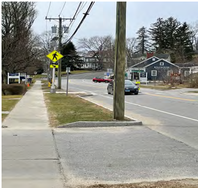
Photo 1: Main Street/Millerton Road
