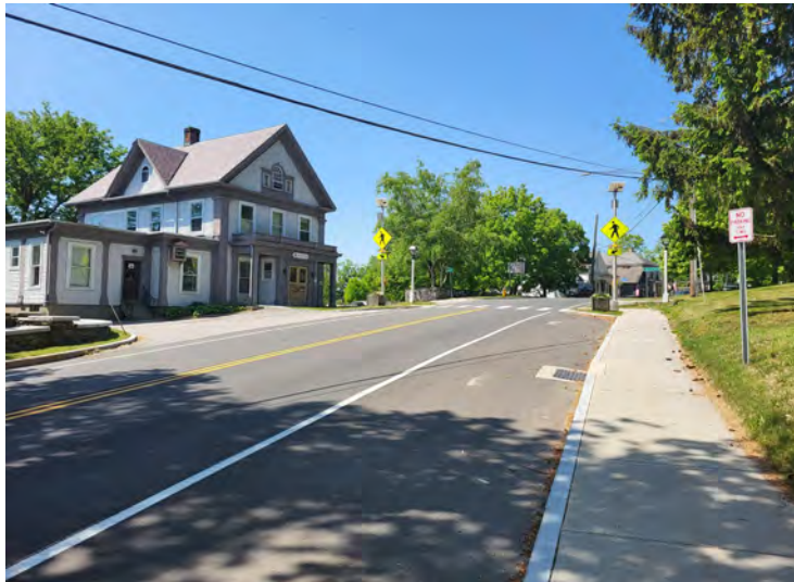
Photo 7: Millerton Road at Holley Street
