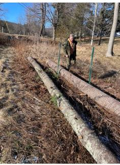
Pine logs for main support of bridge, 2 logs together spaced 6' apart – width of tractor tires. Drawing above indicates diagonal cross beams 6'' x 6'' pressure treated, 8' long on the underbelly of the bridge. Not visible.
