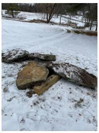
These are the rocks that will support to pine poles to prevent rotting. There will be no concrete or drilling.
