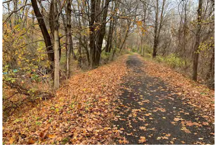
Figure 16: Porous paved portion of Rail Trail
