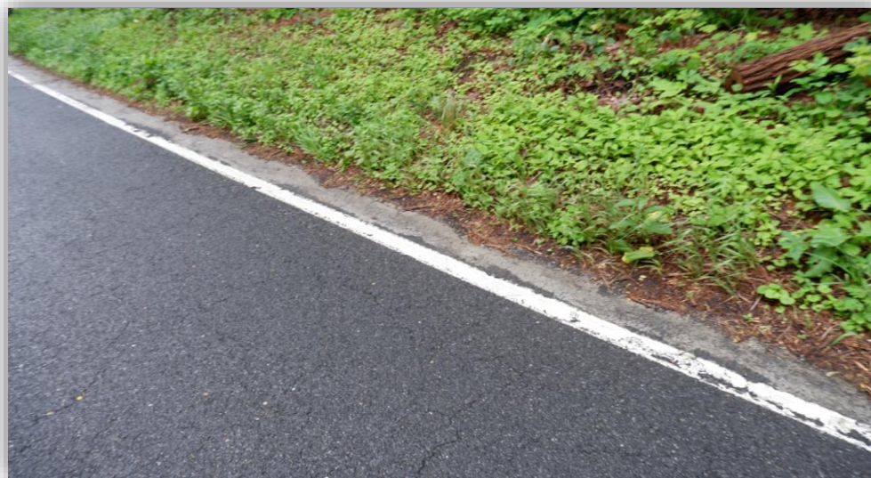
Image 8: Shoulders on CT 41 (Sharon Road) near The Hotchkiss School at North Road less than 1-foot wide
