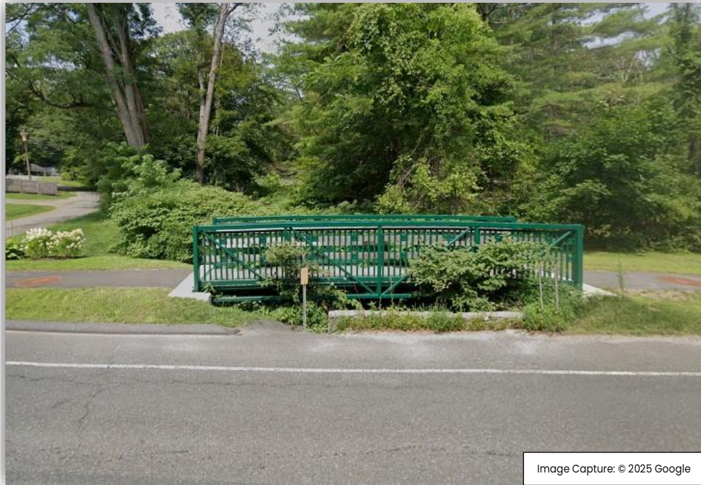
Image 1: CCGP funded pedestrian bridge on the north side of US 44/CT 41
