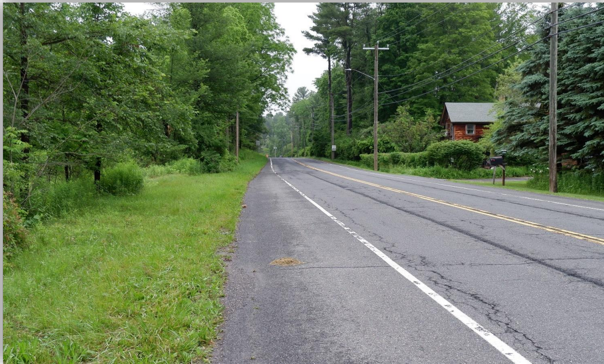
Image 2: CT 41 facing north towards Lakeville center, displaying narrowing shoulder width and lack of sidewalk.
