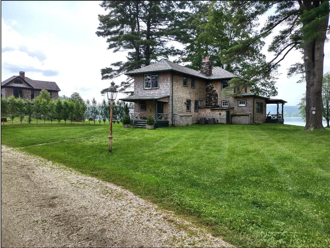
Existing house where addition will be constructed
