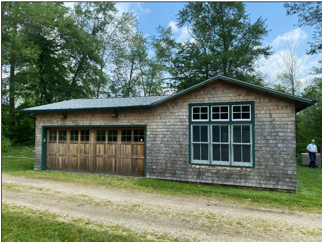
Existing garage to have second story added
