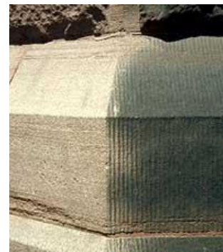
On the left, grit blasting has obliterated the vertical tooling marks from granite, a very dense stone. Photo: NPS files.
