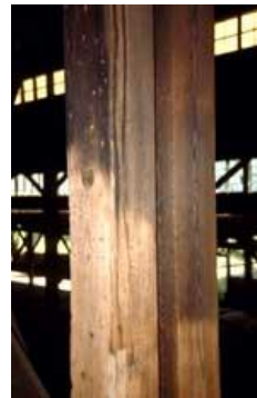
Industrial interiors that are not finely milled may be abrasively cleaned, in some instances. Photo: NPS files.
