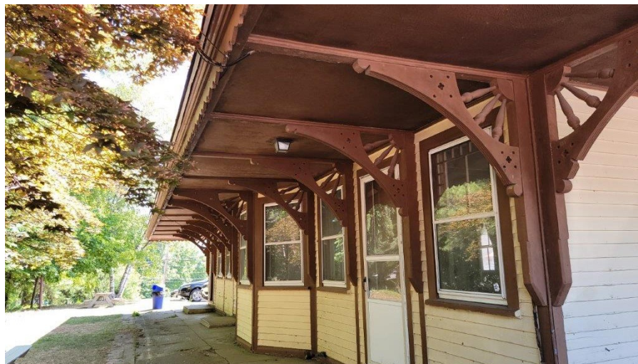
2. North wall of station showing 8 foot overhang and brackets.
