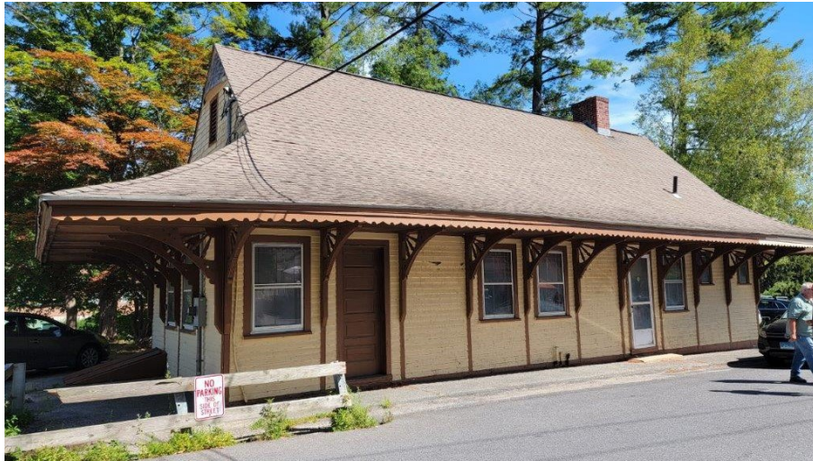
1. South elevation of Lakeville Railroad Station
