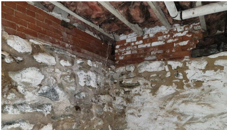
8. Southeast corner of stone foundation with brick on top of wall.
