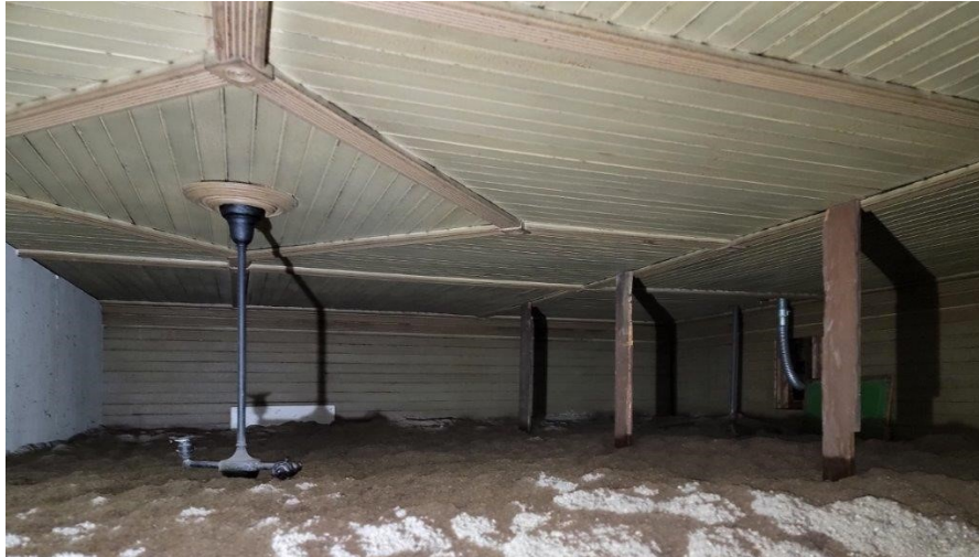
16. Original ceiling and light fixture remains above dropped ceiling.
