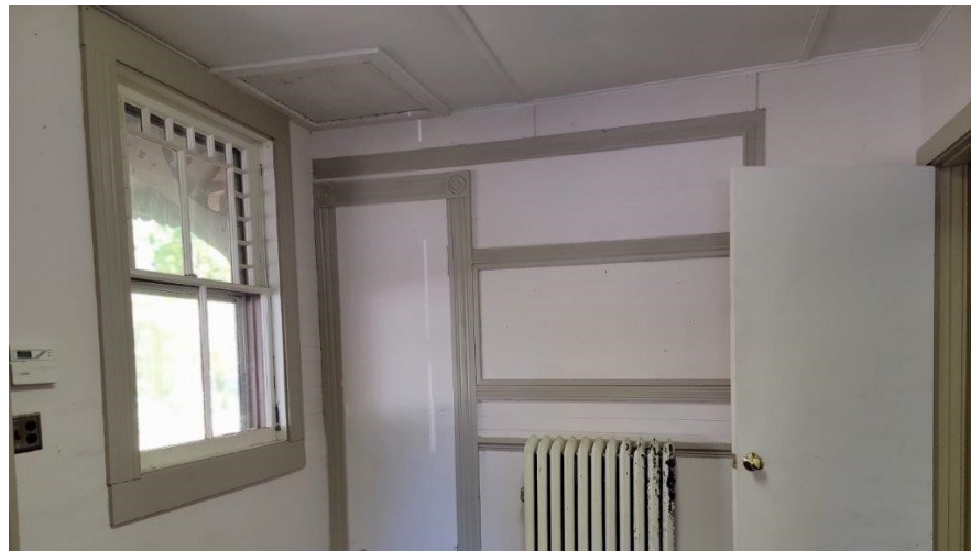
15. Access panel to space above dropped ceiling is in the corner.
